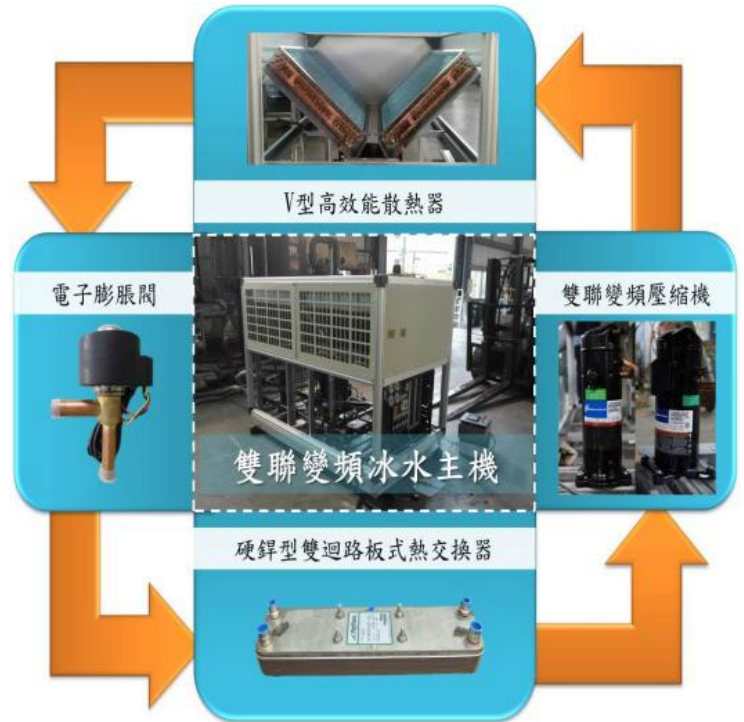
Figure 2. High IPLV and high COP joint dual-inverter chiller
