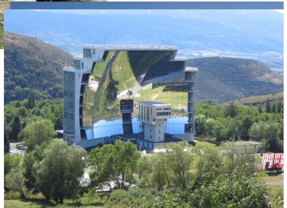
Odeillo solar furnace in France (4000°K)
