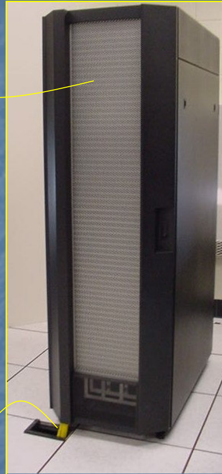
Row of racks (rear) with rack mounted heat exchangers
